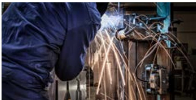
Welding of frame
